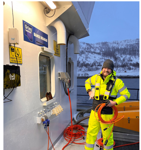
Kristian Kasin Nordlie (WSense) mounting the Gateway on the barge.
